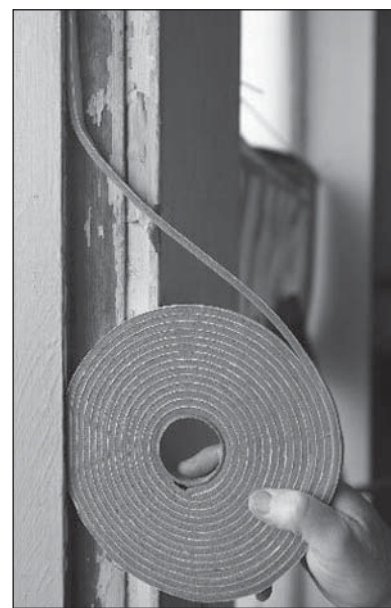
Weather stripping is a quick and cheap way to make your home more comfortable.
